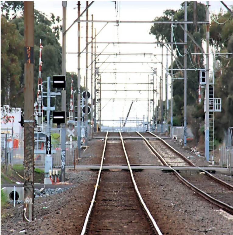
More photos from the resignalling associated with the provision of the single line viaduct between through Bell and Preston. (Above left) The Down outer Home signal protecting the single line, TBY166, is situated well south of Thornbury. Although the Home is situated in roughly the same location as a previous Automatic, the sighting of the Home is badly obstructed by the overhead structures. A banner indicator, TBY166BI, is consequently provided on dead straight piece of track. (Below) Another view of Home TBY166/Banner Repeater TBY166BI with the road set through the single track section, but the with entry Home into the section at stop. If the Signaller had only set the route into Thornbury platform, but not into the single track section, Home TBY166 would show Medium Speed Warning. (Above right) The new style of signal post telephones that are appearing around the Metropolitan area. (Photos: Andrew Waugh)
