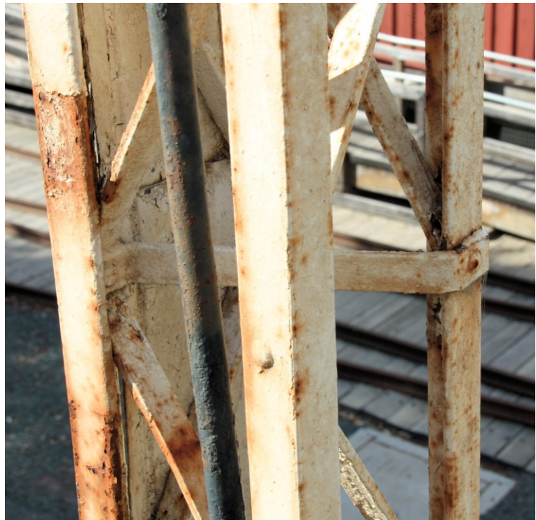
Figure 8 (above). A diagonal brace. Echuca Wharf. The front of the post is to the left. Figure 9 (below). The galvanised iron sheeting on the Up Home from the Tocumwal line at Strathmerton. Note the diagonal brace secured to the front of the angle just above the fishplate on the left angle.
