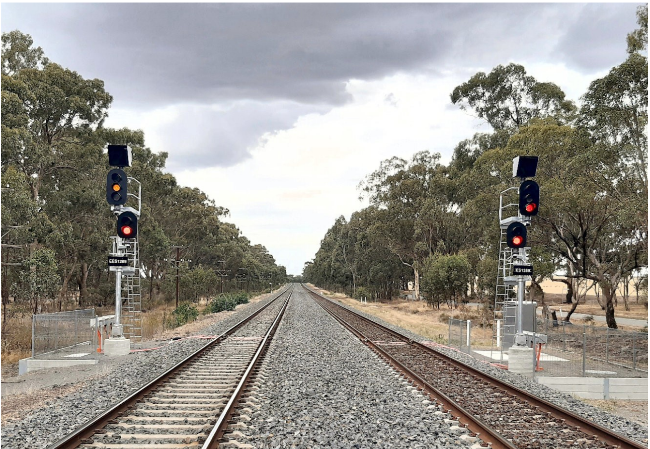
David Langley has sent in some pictures of the new signals at the newly commissioned Longwood crossovers on the North Eastern line. Both photos are taken looking in the Down direction; the upper photo past Homes LWD4 and LWD14, and the lower past Automatics EES1289 and ES1289. In each case the left track is the West Line (former broad gauge) and the right track the East Line.
