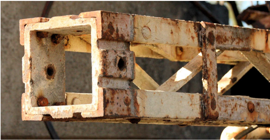
Figure 2. Detail of the distance piece and top of mast, Healesville.
