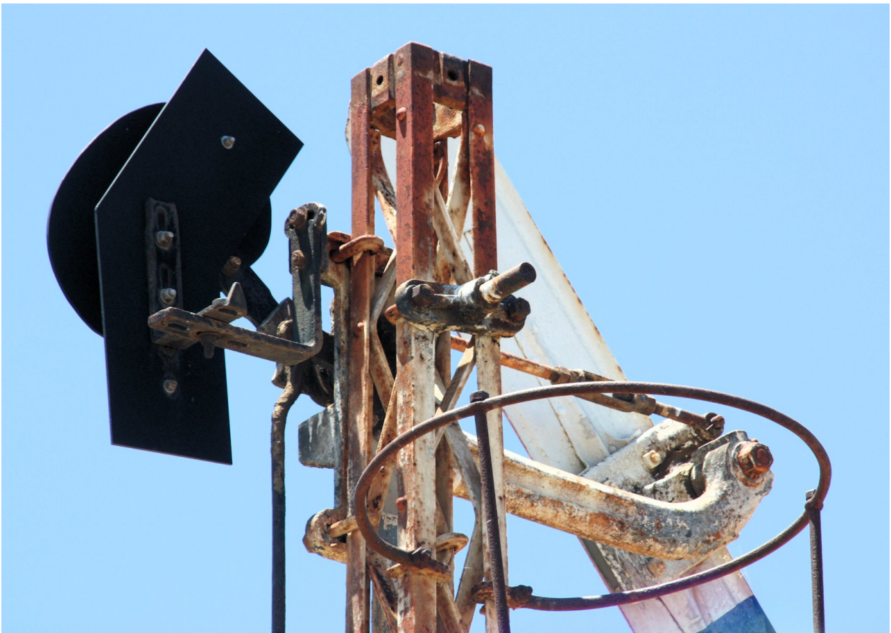
Figure 3. Detail of the rear of the top of the Up Home from the Deniliquin line at Barnes.
