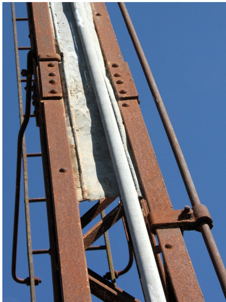
Figure 8 (above). A diagonal brace. Echuca Wharf. The front of the post is to the left. Figure 9 (below). The galvanised iron sheeting on the Up Home from the Tocumwal line at Strathmerton. Note the diagonal brace secured to the front of the angle just above the fishplate on the left angle.
