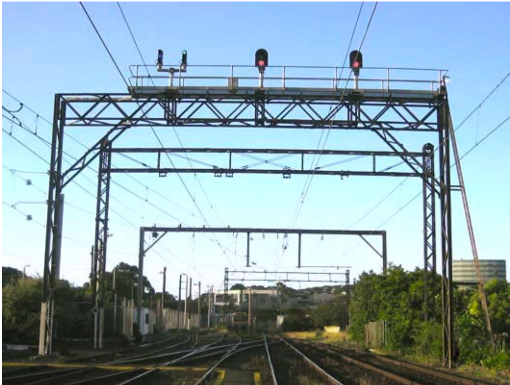
The signalbridge at the Down end of Frankston with the mechanical homes on Posts 13 and 14 replaced by light signals, and the Discs on Post 12 replaced by a 'bracket' post with two Dwarf signals. Photo: Keith Lambert
