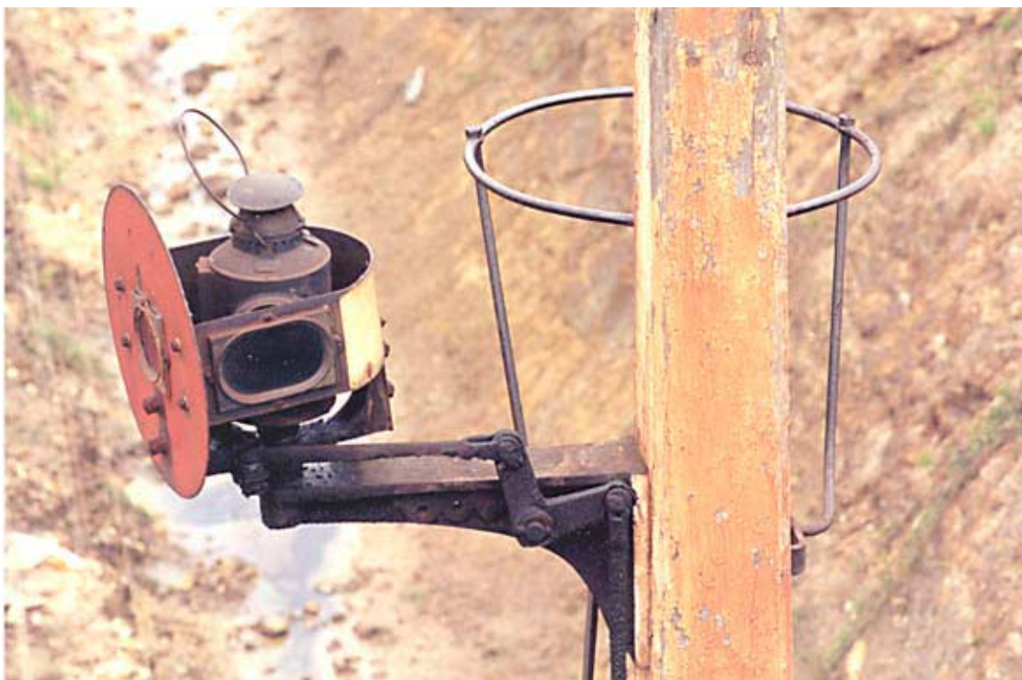
Disc 13" turned off" for the locomotive of a Down passenger train to run around its train. The disc has not come fully off due to insufficient travel in the connection to the signalbox, but the intention is clear and at night the elongated green lens would give a clear signal at night. The arrangement of the downrod, crank, and operating rod can be clearly seen. The disc was oil lit and the lamp can be seen in the centre of the target.
