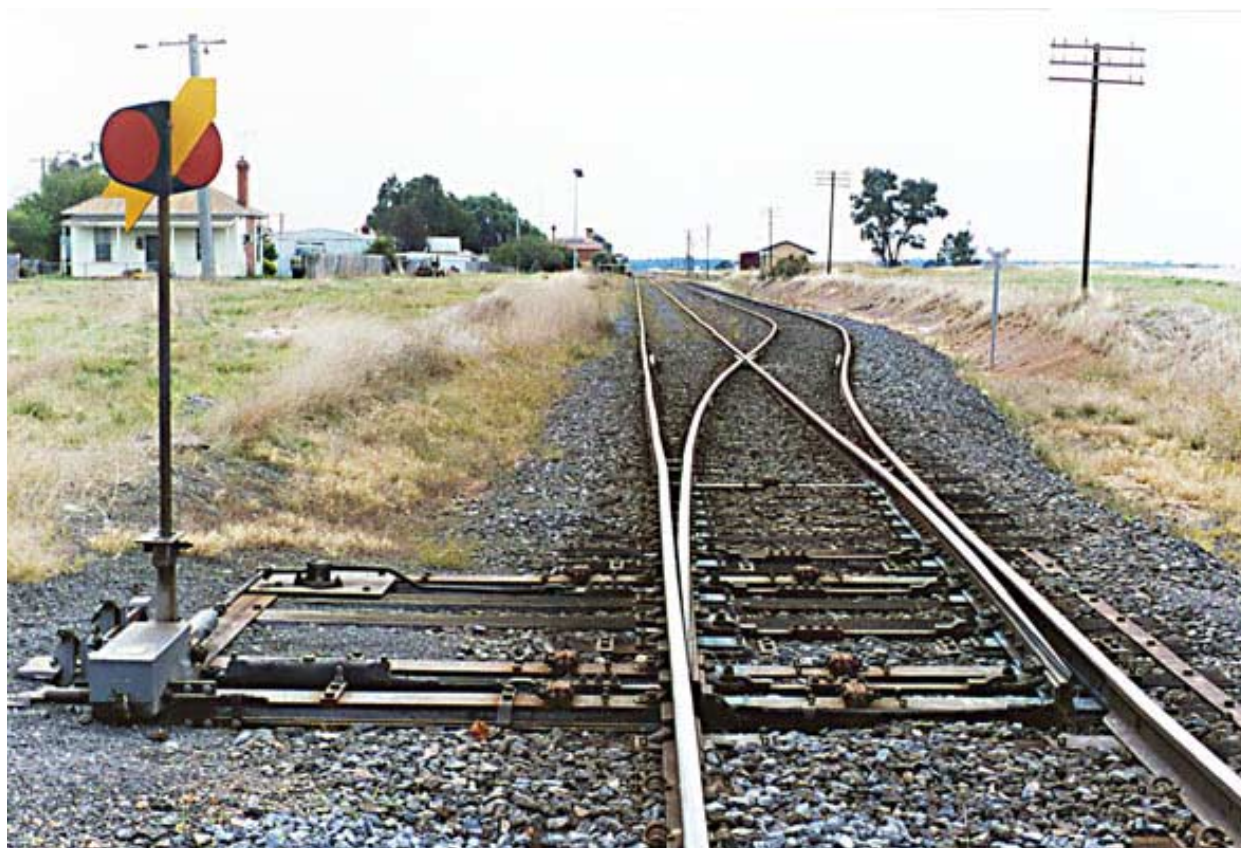
(Left) The assembly drawing for the Victorian dwarf switchstand H620. This was produced for use where a switchstand had to be located between two tracks and, as far as is known, was only used at the Up end of Moe. The drawing is dated 18 October 1930 and no amendments have been subsequently made. (Above) The Down end trailable points at Carwarp on the Mildura line. The trailable points on this line are equipped with switchstands that show an arrow when the points are set and locked for a train to arrive. The loops are arranged so that Up trains (i.e. loaded grain trains) arrive into the straight road. Straight moves are indicated by a green arrow, as shown here. Down trains arrive into the loop and this is indicated by a yellow arrow. (Below) The Up end trainable points at Talbot, again on the Mildura line. The trailable point machines on this line are Westinghouse Type S21M which were developed from the US&S Type S21 machines. These machines can be trailed at speeds up to 80 km/h. The banner indicates the position of the plunger lock and when plunger is withdrawn from the lockbar shows two red discs - as was occurring at Talbot when this photo was taken.
