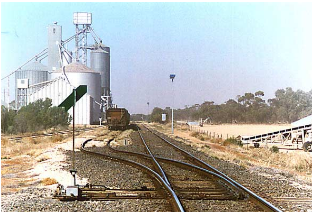
(Left) The assembly drawing for the Victorian dwarf switchstand H620. This was produced for use where a switchstand had to be located between two tracks and, as far as is known, was only used at the Up end of Moe. The drawing is dated 18 October 1930 and no amendments have been subsequently made. (Above) The Down end trailable points at Carwarp on the Mildura line. The trailable points on this line are equipped with switchstands that show an arrow when the points are set and locked for a train to arrive. The loops are arranged so that Up trains (i.e. loaded grain trains) arrive into the straight road. Straight moves are indicated by a green arrow, as shown here. Down trains arrive into the loop and this is indicated by a yellow arrow. (Below) The Up end trainable points at Talbot, again on the Mildura line. The trailable point machines on this line are Westinghouse Type S21M which were developed from the US&S Type S21 machines. These machines can be trailed at speeds up to 80 km/h. The banner indicates the position of the plunger lock and when plunger is withdrawn from the lockbar shows two red discs - as was occurring at Talbot when this photo was taken.
