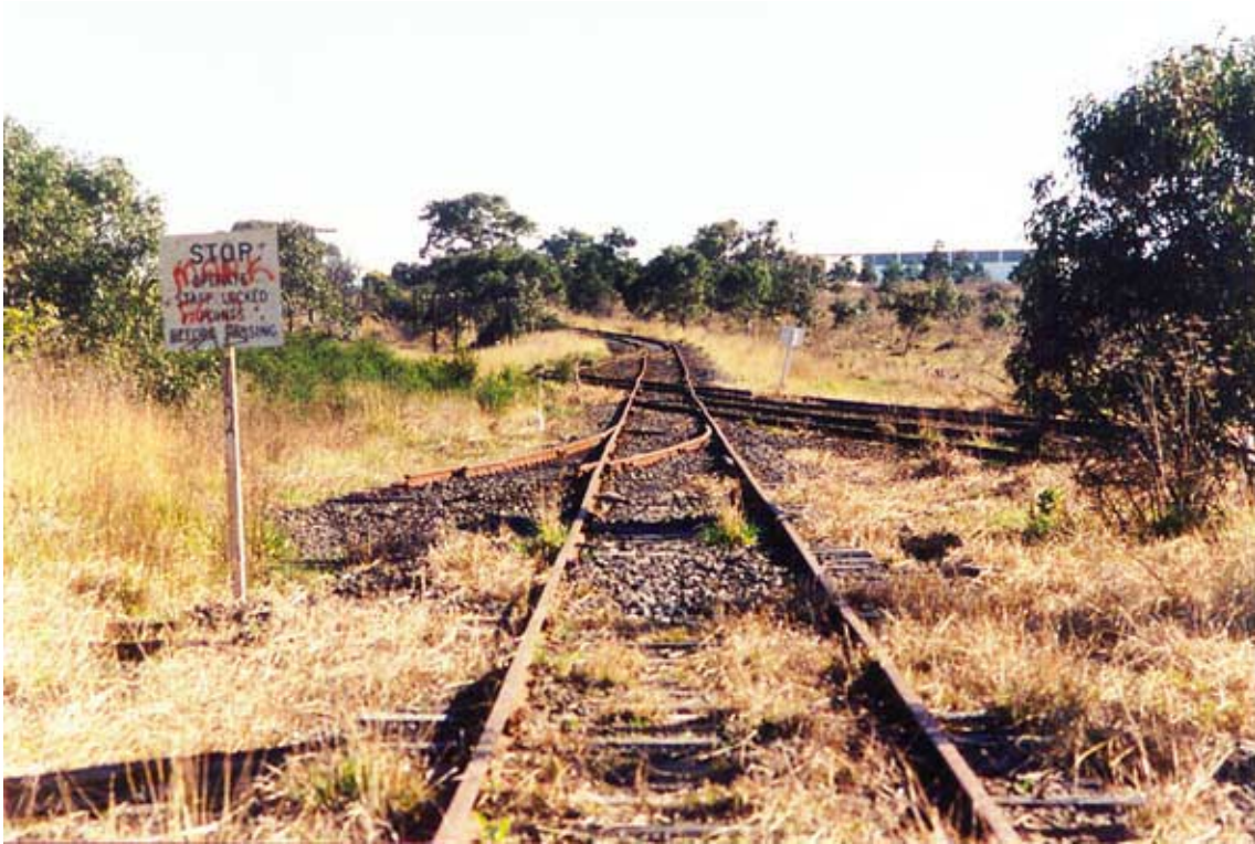
Ford's Siding looking in the Down direction in September 1994. The Ford's Sidings themselves are behind the camera on the right, and the broad and standard gauge leads to the sidings can be seen coming in from behind the clump of trees. The Standard Gauge line is the furthest siding and it can be seen how this crosses the Broad Gauge 'main' line at a diamond crossing before swinging back to become the Dual Gauge track to Somerton just at the start of the curve in the distance. The points in the foreground led to the Tubemaker's Siding, but this siding had been lifted at the date of the photo. The Union Steel Siding leads from the Standard Gauge line adjacent to the diamond crossing.
